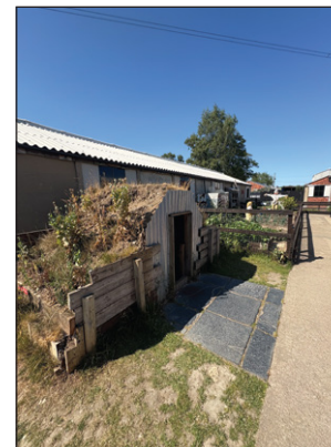
A photo of an air raid shelter which was designed to keep people safe during German air attacks.
