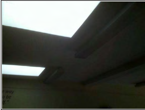
Ceilings: Plasterboard to wooden joists
