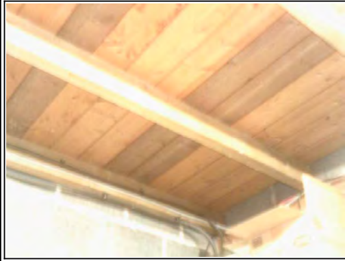
Ceilings: Wood boards
