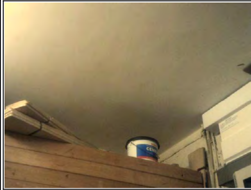
Ceilings: Plasterboard to wooden joists
