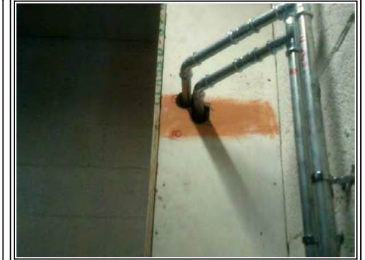
Other: Wood boxing to pipework
