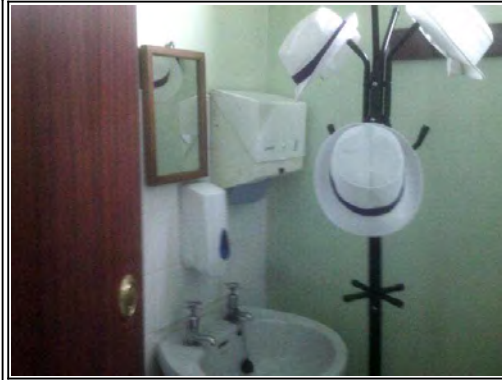
Walls: Solid masonry with plaster skim partly ceramic tiled
