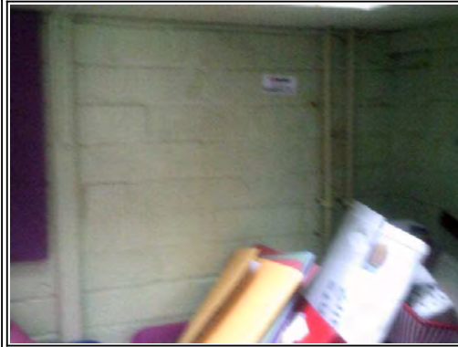
Walls: Solid Brick
