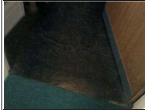
Floors: Concrete beneath floor tiles
