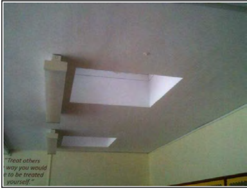
Ceilings: Plasterboard to wooden joists
