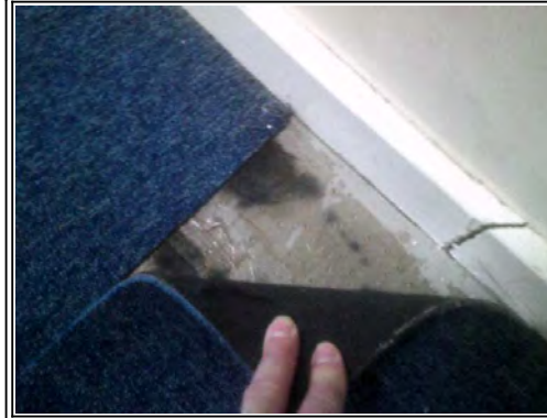
Floors: Concrete beneath carpet
