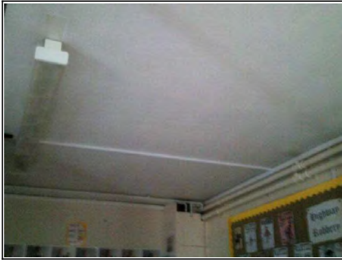
Ceilings: Plasterboard to wooden joists
