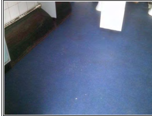
Floors: Concrete beneath vinyl
