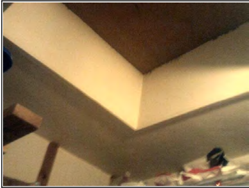
Ceilings: Plasterboard to wooden joists
