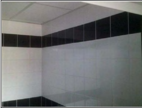
Walls: Solid masonry behind ceramic tiles
