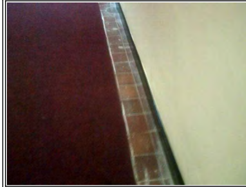
Floors: Quarry tiles beneath carpet
