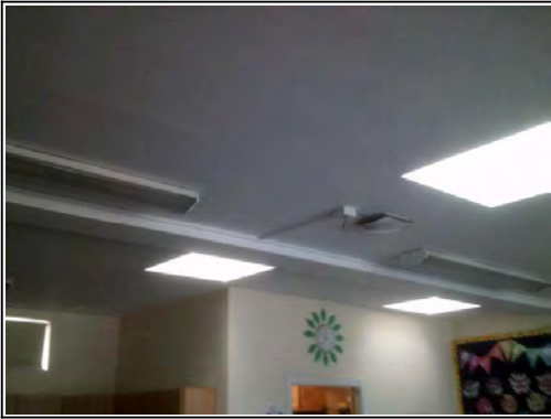
Ceilings: Plasterboard to wooden joists
