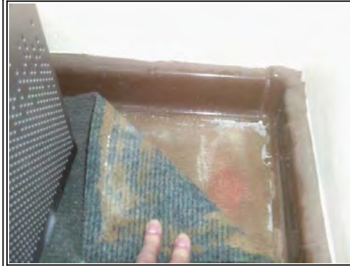
Floors: Quarry tiles beneath carpet
