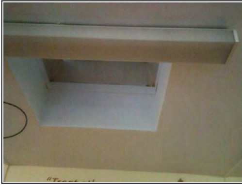
Ceilings: Plasterboard to wooden joists
