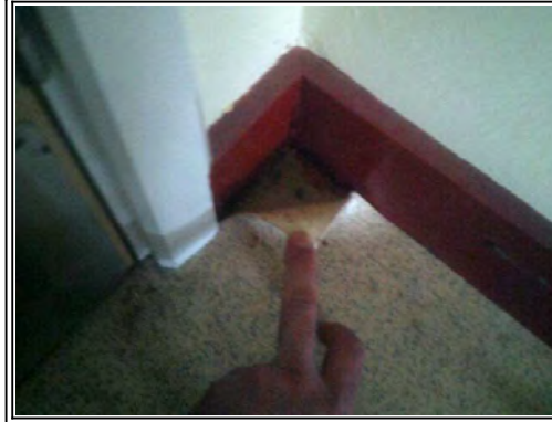
Floors: Floor tiles beneath carpet and vinyl
