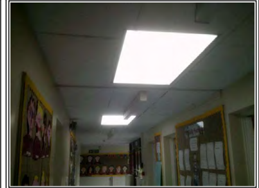
Other: Negative skylight
