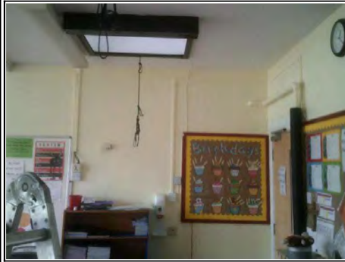
Walls: Solid masonry with plaster skim
