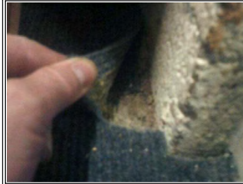
Floors: Concrete beneath floor tiles and carpet
