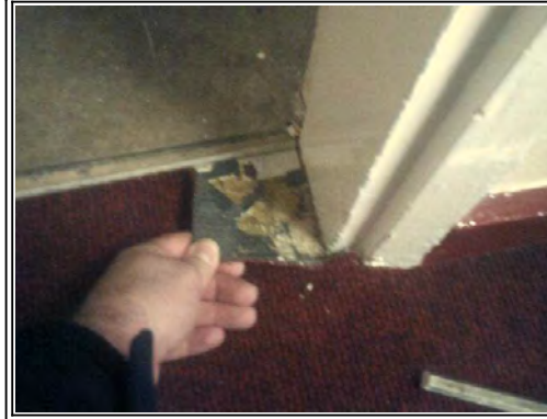
Floors: Floor tiles beneath carpet and vinyl
