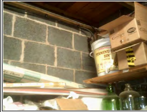
Walls: Solid Block
