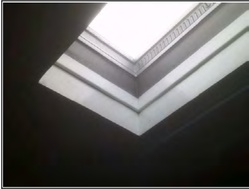
Ceilings: Plasterboard to wooden joists
