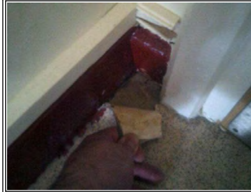
Floors: Floor tiles beneath carpet and vinyl
