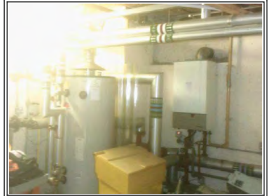
Other: Negative plant and pipework. Negative electrics.
