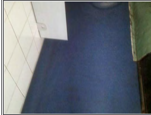
Floors: Concrete beneath vinyl
