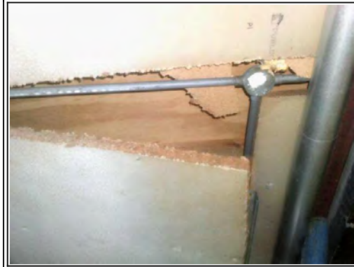
Ceilings: Wood above foam insulation
