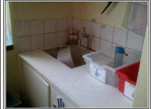
Other: Negative sink unit and negative skylights
