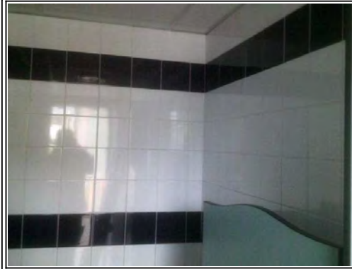
Walls: Solid masonry behind ceramic tiles
