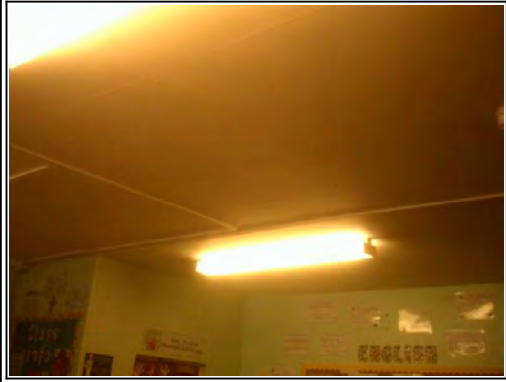
Ceilings: Plasterboard to wooden joists
