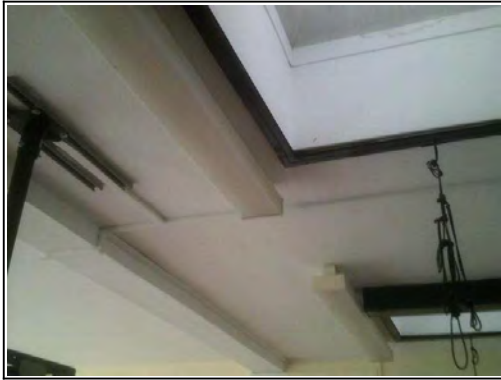
Ceilings: Plasterboard to wooden joists
