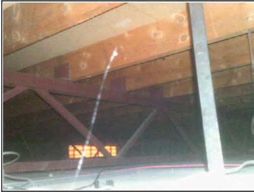
Ceilings: Wood above suspended ceiling
