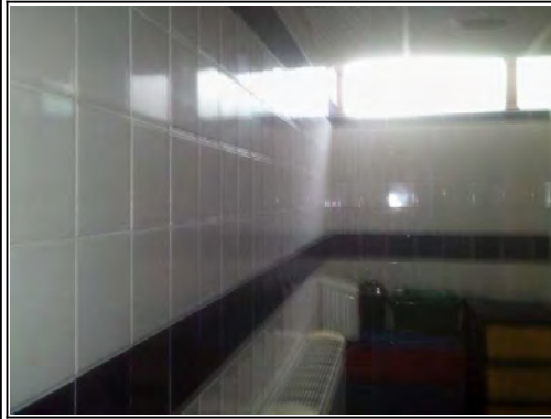
Walls: Solid masonry behind ceramic tiles
