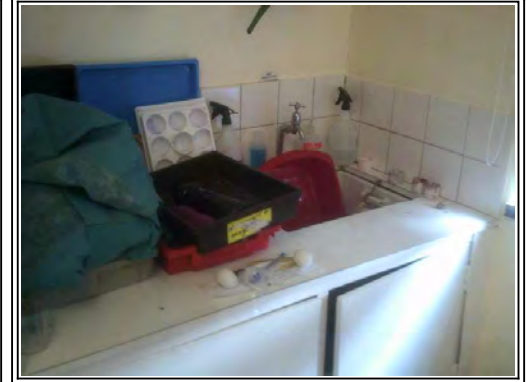
Other: Negative sink unit and negative skylights
