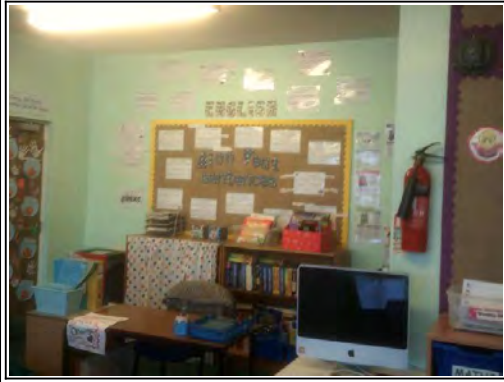
Walls: Solid masonry with plaster skim
