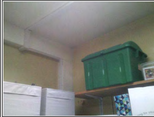
Walls: Solid masonry with plaster skim
