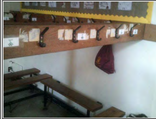
Walls: Solid masonry with plaster skim
