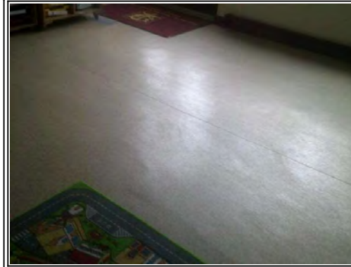
Floors: Concrete beneath vinyl
