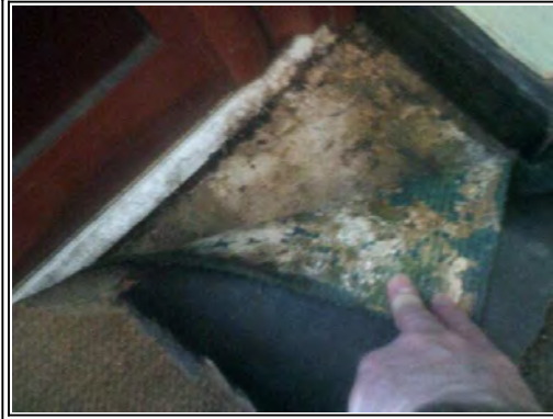
Floors: Concrete beneath carpet
