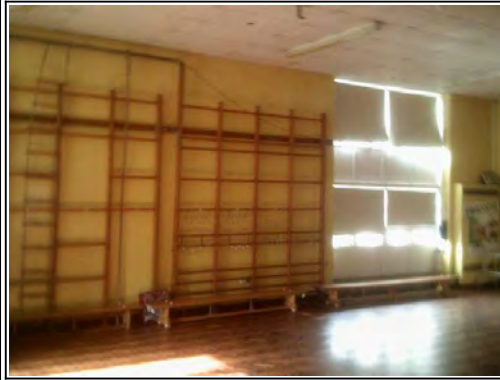
Walls: Solid masonry with plaster skim
