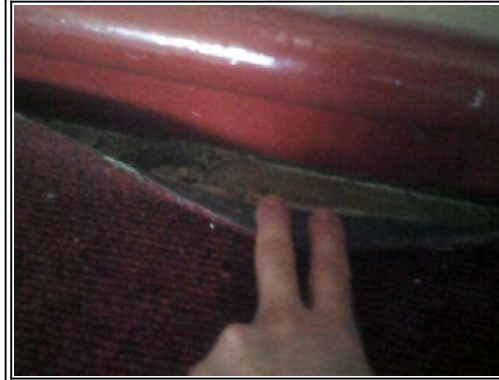
Floors: Floor tiles beneath carpet and vinyl
