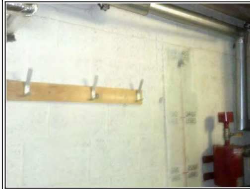
Walls: Solid Block
