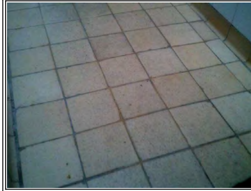
Floors: Ceramic tiles partly beneath carpet
