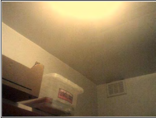
Ceilings: Plasterboard to wooden joists
