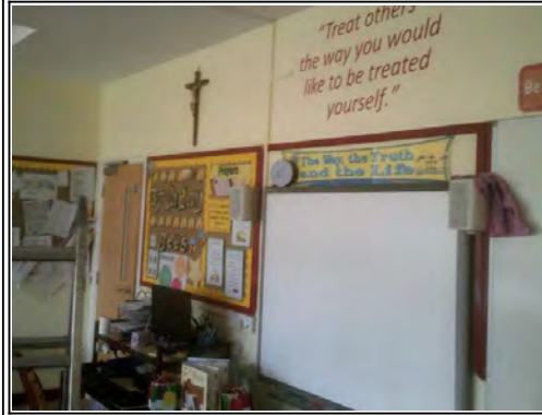
Walls: Solid masonry with plaster skim
