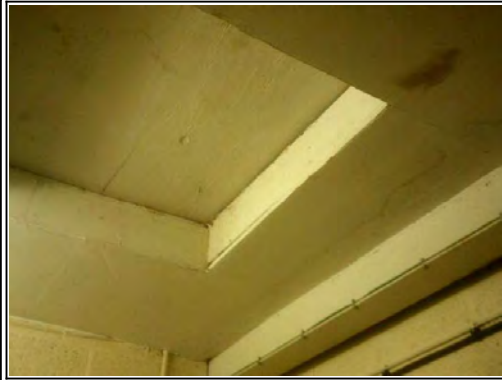
Ceilings: Plasterboard to wooden joists
