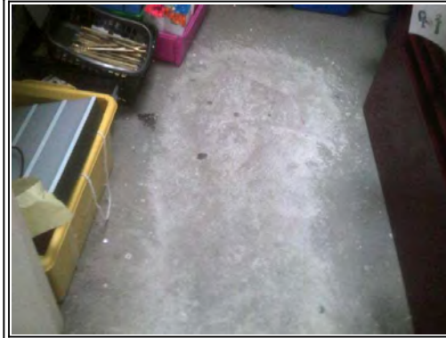
Floors: Concrete beneath vinyl
