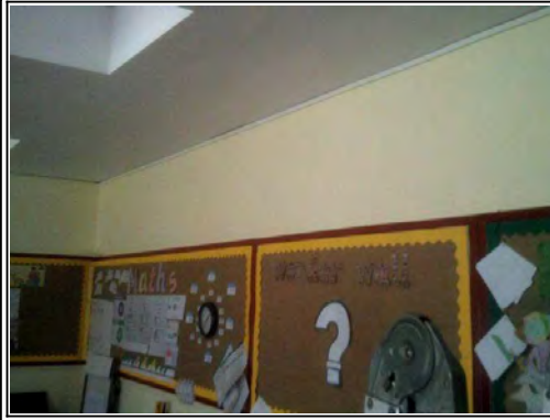
Walls: Solid masonry with plaster skim
