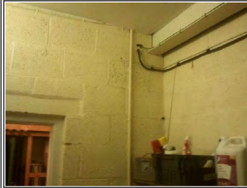
Walls: Solid Block
