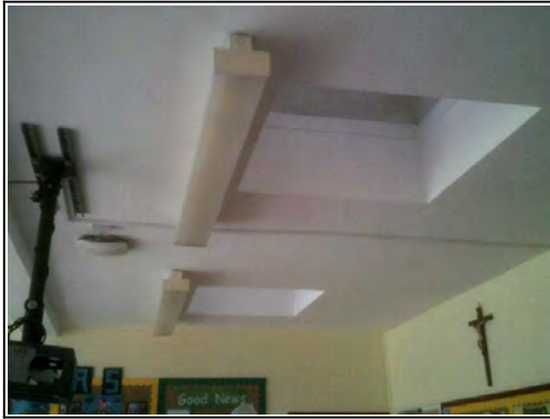
Ceilings: Plasterboard to wooden joists
