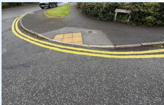
It is illegal for cars to stop alongside the dropped curbs
