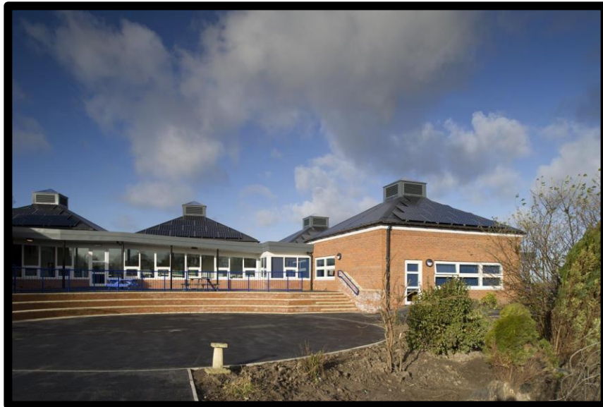
The extension to the rear which was added in 2011
